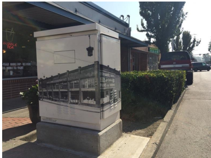
Utility box with vinyl wrapping in Downtown Renton (City of Renton)
